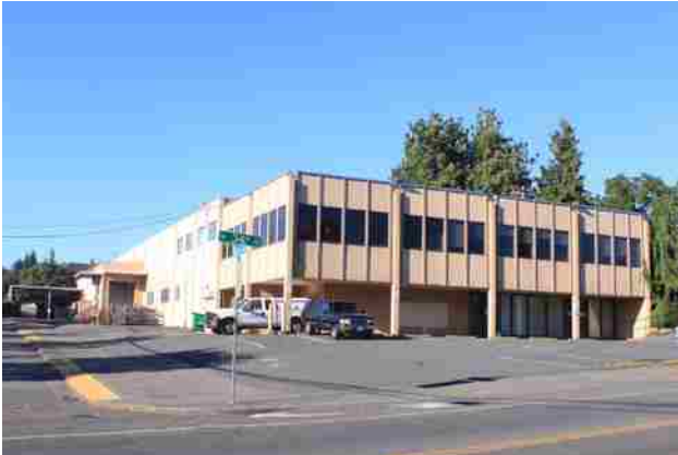
Fig. 3.9 Exterior view of the existing SPU warehouse
