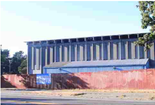
Fig. 3.1 Existing Seattle North Solid Waste Transfer Center
