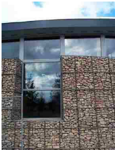
Fig. 2.3 The Earth Center, Doncaster, UK, Bill Dunster
